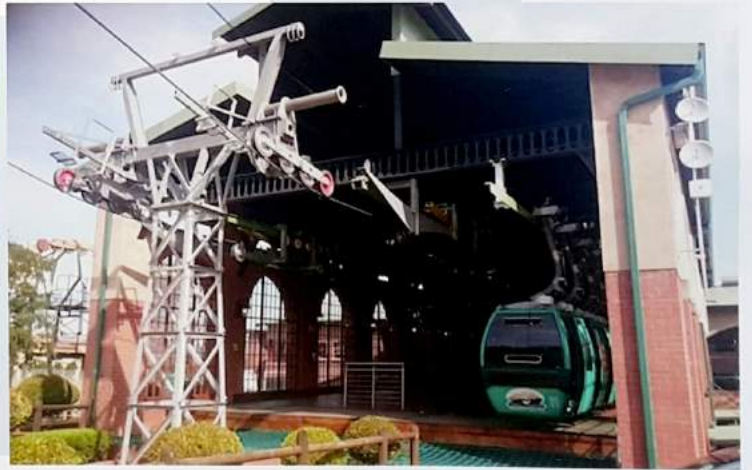
EXAMPLES OF DRIVE STATION ASSEMBLY
