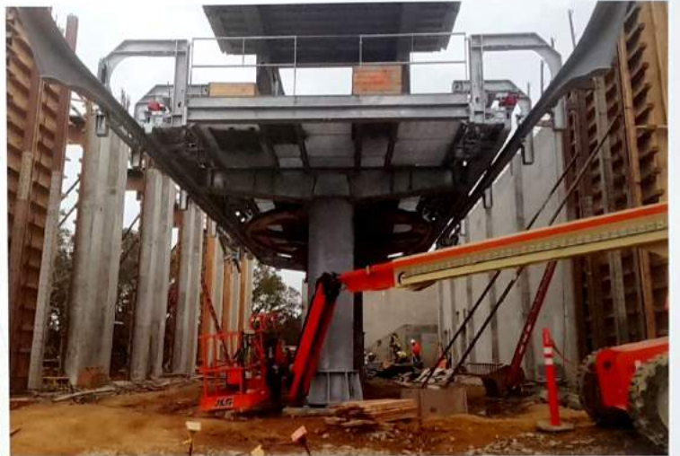
EXAMPLES OF DRIVE STATION ASSEMBLY
