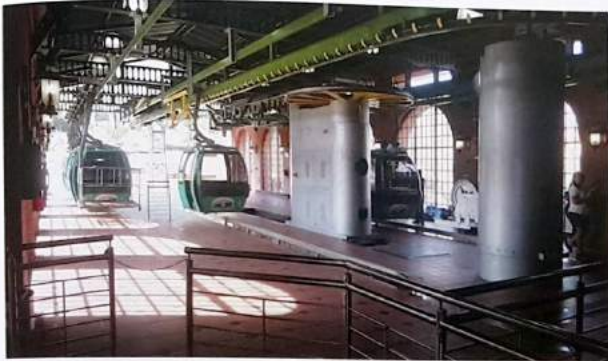
BASE STATION AT HARTBESPOORT CABLE WAY, SOUTH AFRICA
